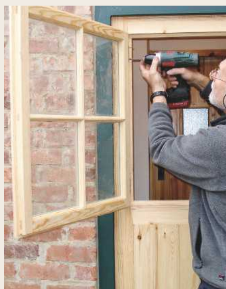
▲ Pic.4 Having fitted the glazing it's time to hang the door...
